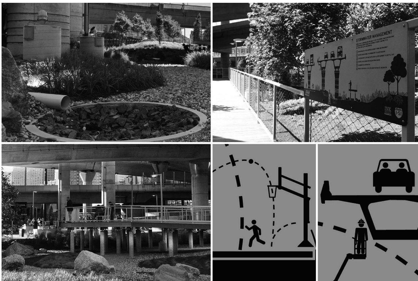
Figure 4: Infra-Space storm-water dissipation basin in the constructed wetland, informational signage of storm-water system, elevated viaduct under the elevated viaduct, basketball/maintenance signage details, 2017
